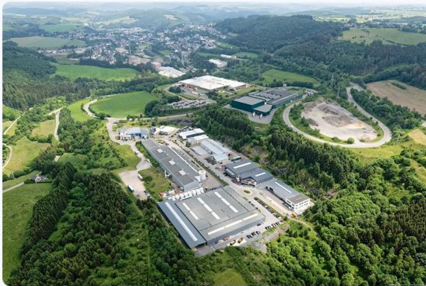
No-Nail Boxes aerial view;
